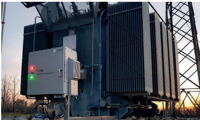
Figure 1. Online holistic monitoring system installed in 25 MVA GSU
