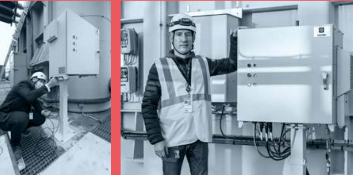
Customer Installation: T1-G5-INT3-TFC+Models: TOTUS with DGA 5 Gas, PD and Bushing Monitoring on 3 bushings with Transformer Models
