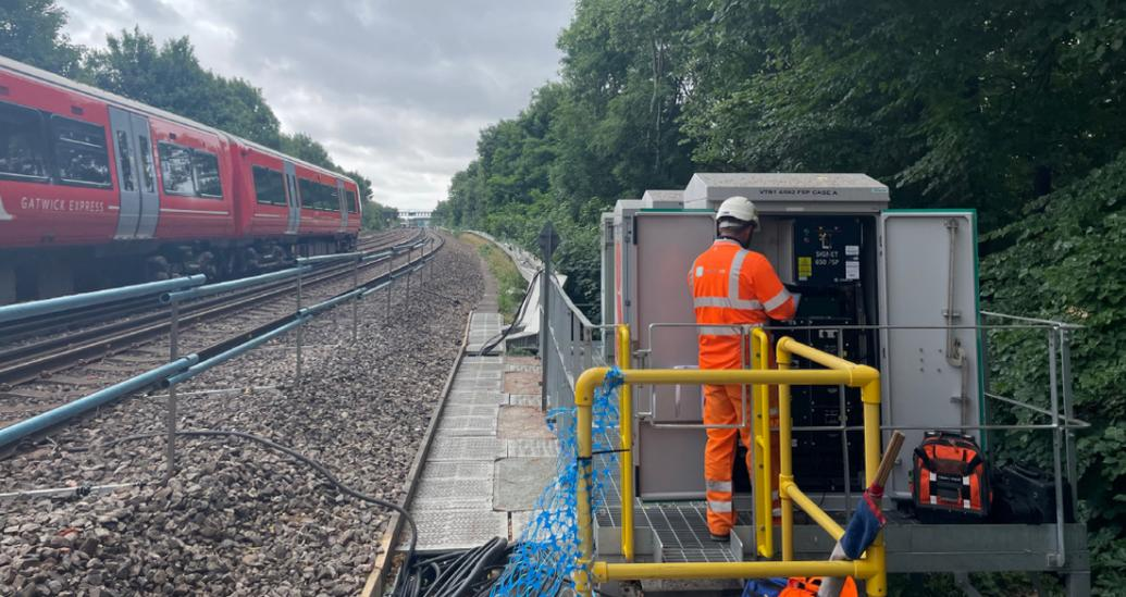
» *"On the West Coast Main line, Signet replaced the traditional LV power supply fuse protection systems to provide coordination and basic sectionalisation which was proving to be expensive and labour intensive and often resulted in long train delays and lost minutes. Signet solves this problem in a cost effective and controllable manner by automatically restoring power to affected signals and reconfiguring the system to isolate the fault."*
